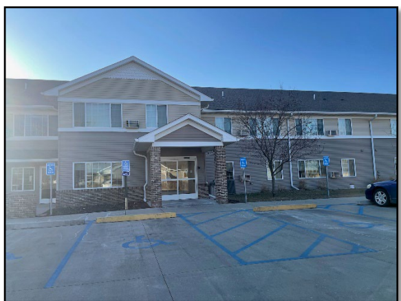
Buffalo Ridge Apartments (Worthington)
